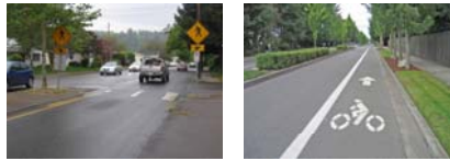
Bicycle and pedestrian infrastructure supporting transit facilities and bus stops
